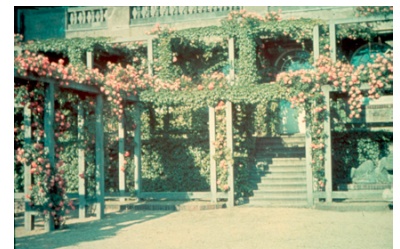
124.2 Pergola of the Exhibition Hall, photo c. 1940
