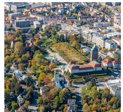
27.2 Mathildenhöhe Darmstadt, aerial view from east, photo 2017
