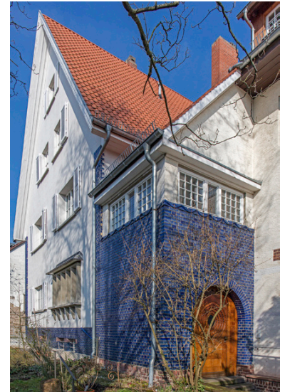
97.1 Joseph Maria Olbrich, Three House Group, Blue House, 1904, view from south-west, photo 2016
