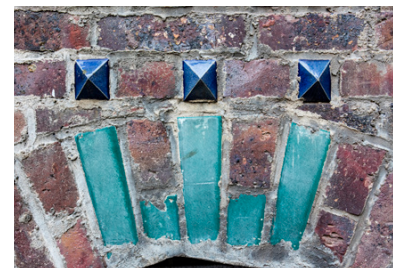
97.2 Joseph Maria Olbrich, Three House Group, Corner House, detail of window lintel, 1904, photo 2016
