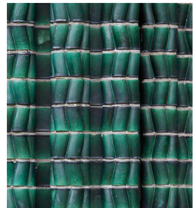
55.1 Peter Behrens, Glazed bricks of the Behrens House, 1901, photo 2013
