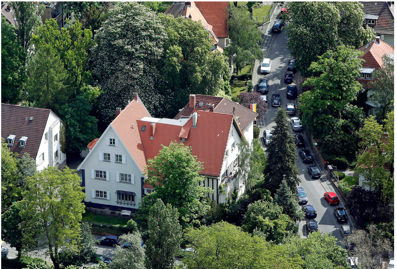
96.1 Joseph Maria Olbrich, Three House Group, 1904, aerial view from south-west, photo 2012
