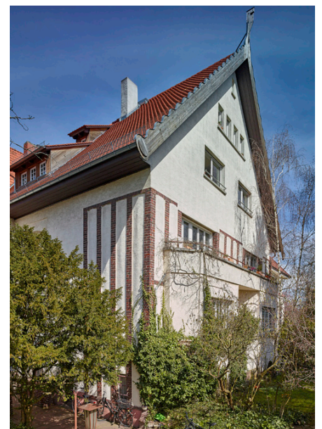
96.4 Joseph Maria Olbrich, Three House Group, Corner House, 1904, view from south-west, photo 2015
