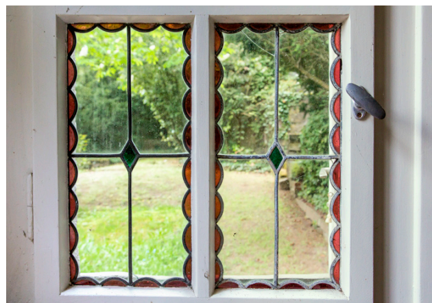
77.3 Jakob Krug, Garden House, 1910, windows, photo 2018
