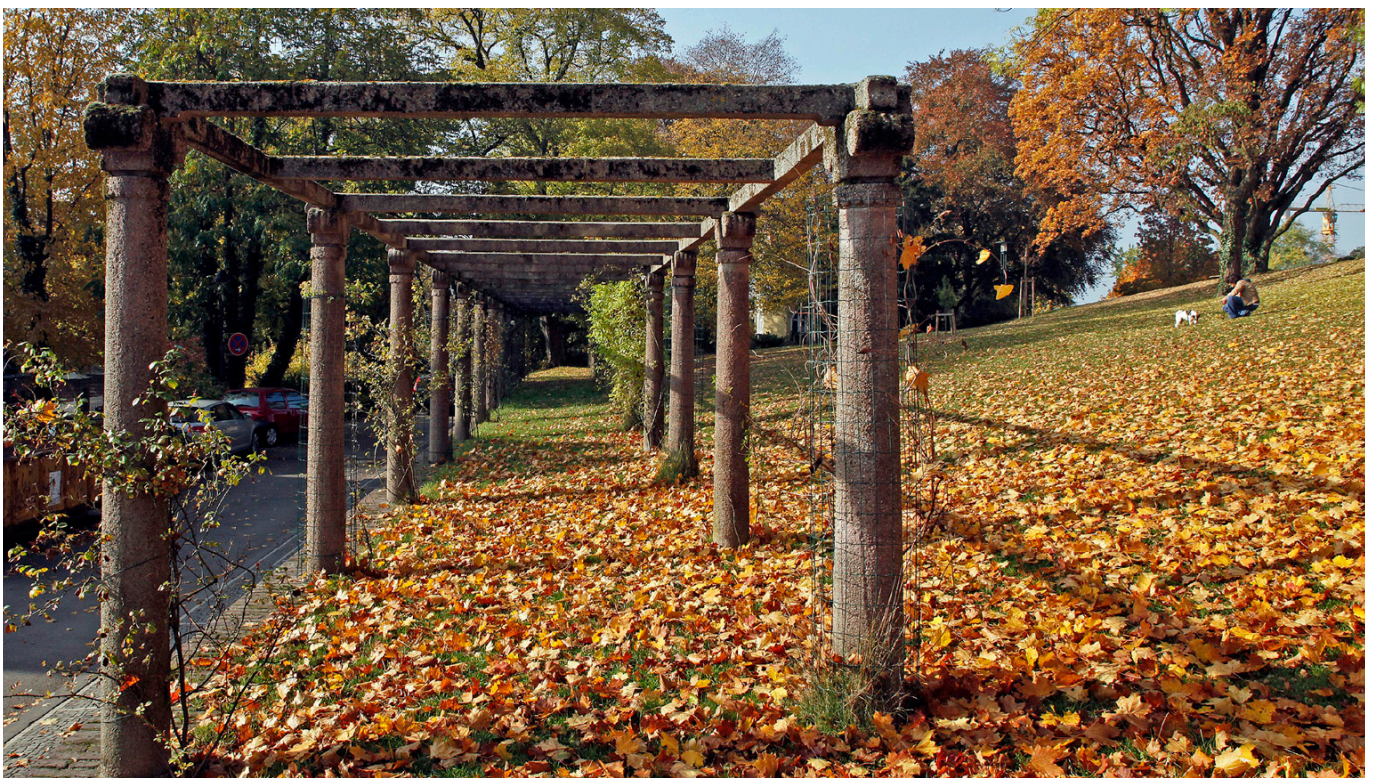
84.2 Albin Müller, Concrete Pergolas, 1914, view from east, photo 2009
