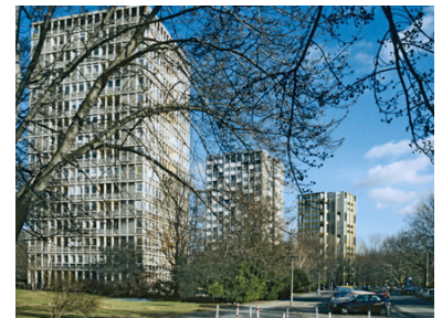
198.2 Hansaviertel, Interbau 1957, High-rise Residential Buildings at Bartning-Allee, Berlin
