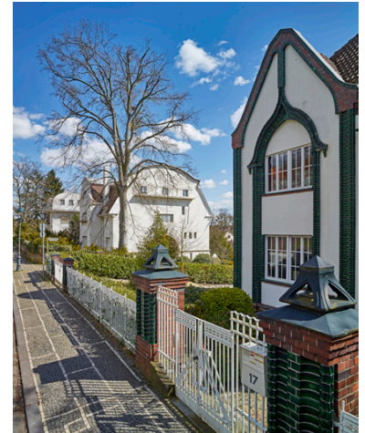
28.1 Peter Behrens and Joseph Maria Olbrich, Behrens House, Large Glückert House and Small Glückert House, 1901, view from west, photo 2015
