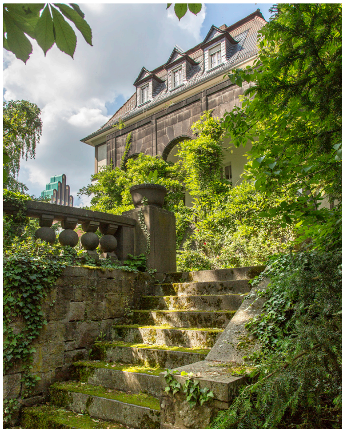
77.1 Upper Hessian House, 1908, view from south-east, photo 2018
